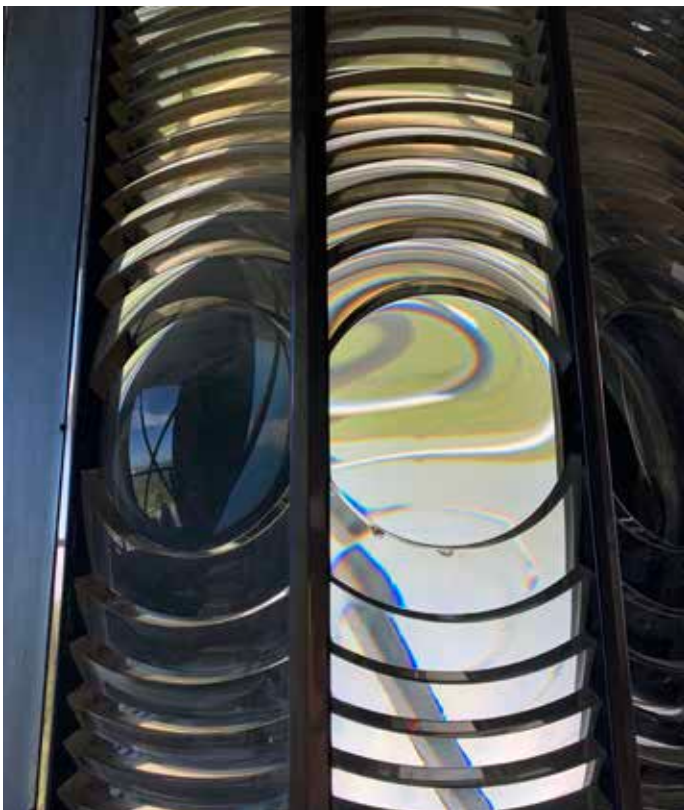
LEFT TOP: The optic viewed in 2021 from the balcony is the original of 1904, although some of the panels have been removed. Notice the diagonal arrangement of the astragals that hold the curved lantern glass in place. Left Bottom: Two of the vertical panels. RIGHT TOP: The bulls-eye lenses offer beautiful reflections by day. RIGHT CENTRE: The mercury bath that supports the weight of the four-ton optic is hidden inside the base. The frictionless rotation is assisted by balance wheels that help to keep the optic in the horizontal plane. RIGHT BOTTOM: The more modern lamp changer with its tungsten filament bulbs replaced the original electric arc equipment in 19xx.
