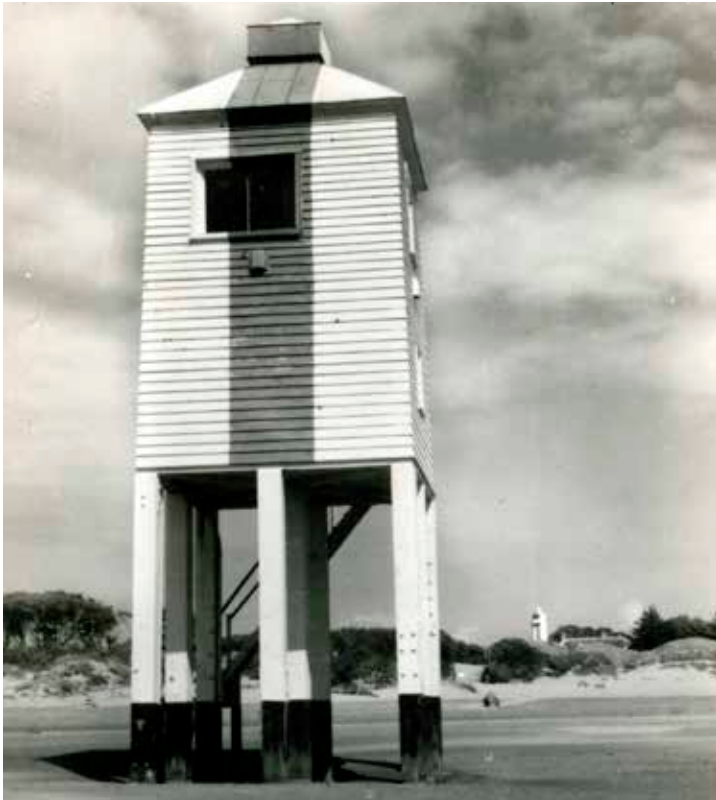
ABOVE: An old photograph of the two leading lights at Burnham-on-Sea. In the foreground, the Low Light is mounted on piles on the beach, whilst the High Light is just visible ashore in the distance.
