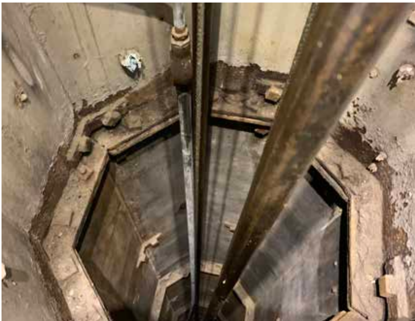
LEFT TOP: The clockwork mechanism that rotated the optic in the lantern of the South Foreland High Light. Like all mechanical clocks, it needed the keepers to wind it, in this case, 100 turns of the winding handle to keep the rotation going for about 2\frac{1}{2} hours. LEFT BOTTOM: The winding of the clock raised a weight suspended on a wire on the inside of a tube at the centre of the lighthouse. As the clock ran down, the weight fell to the bottom whereupon it was time to wind it back up to the top. RIGHT TOP: The octagonal tube containing the clock weight occupies the centre of the tower and predominates in the lower room of the lighthouse. RIGHT BOTTOM: The tube is also present in the service room (below the lantern room), of course, where a bell is mounted so as to give warning to the keepers when the clock needs to be rewound.
